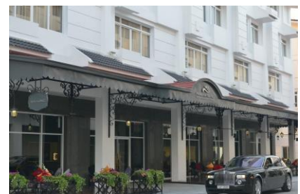
PARADISE SUITES HOTEL, HALONG BAY
